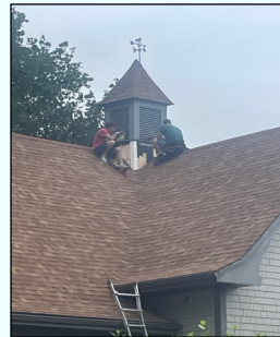
Carriage House Cupola leak being repaired.
