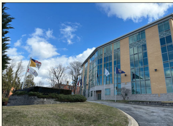
Residence and offices, Archdiocese for the Military Services, USA. Washington, D.C.
